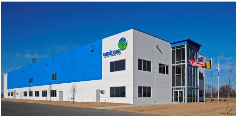
Picture : Side view of Umicore’s new facility for germanium wafers in Quapaw, OK, USA.
